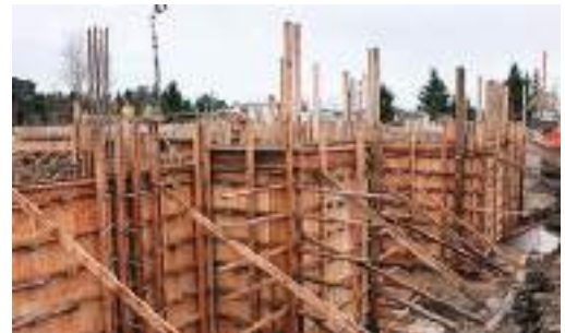
Fig. 4.4 (a): Shuttering for beam and RCC Floor
