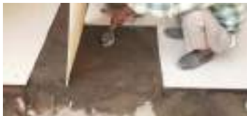
Step 2: Pasting of mortar
