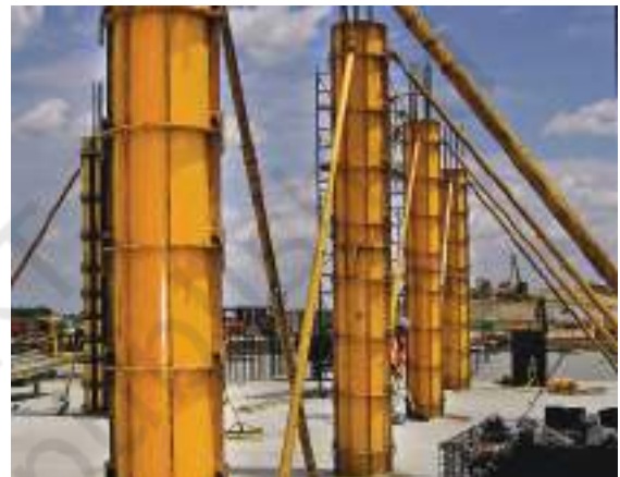
Fig. 4.2: Formwork for circular columns
