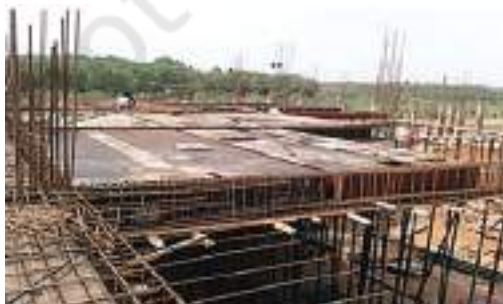
Fig. 4.4 (a): Shuttering for beam and RCC Floor
