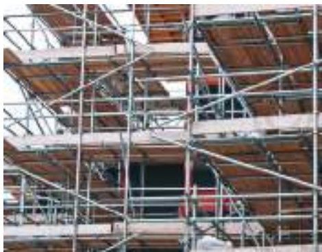
Fig. 3.7: Cantilever Scaffolding
