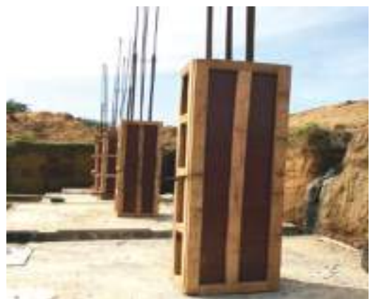
Fig. 4.3: Formwork for square or rectangle columns
