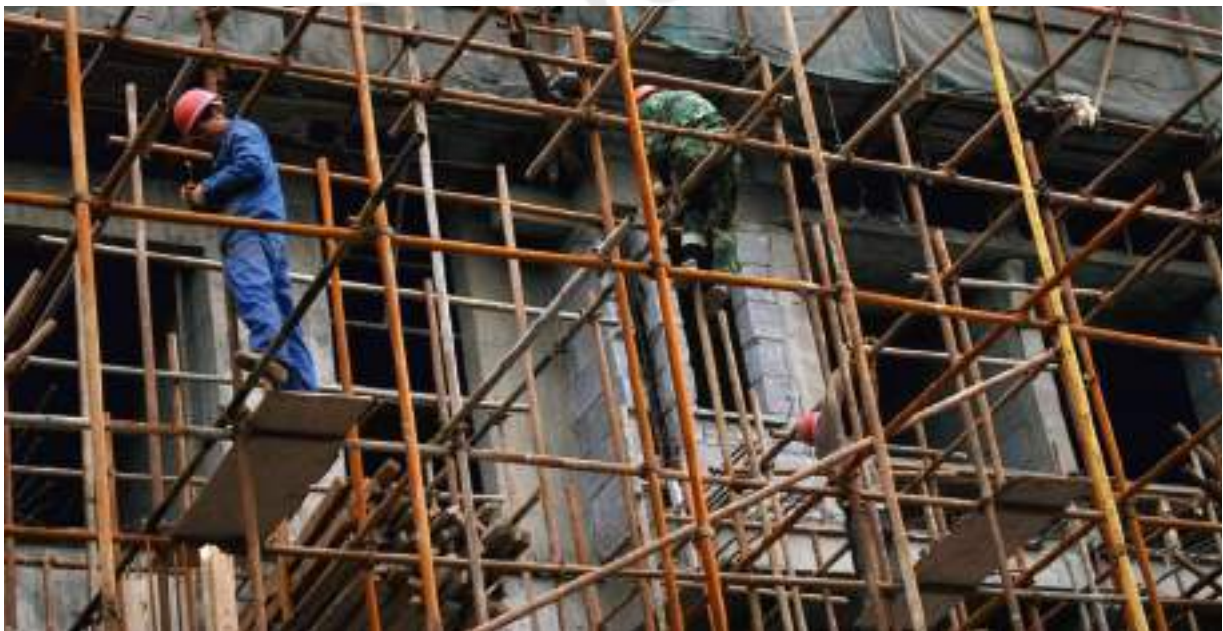
Fig. 3.1: A view of Scaffolding
