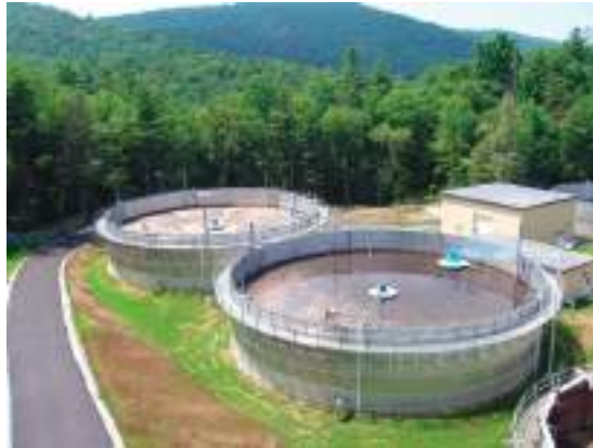
Fig 16. Sequential batch reactor (SBR)
