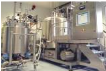
Figure 4.21 Maintenance of Process Equipments
