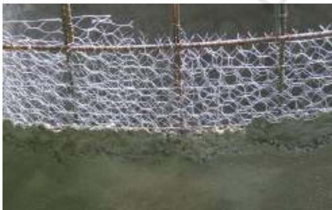
Fig.2.23: Ferro Cement work
