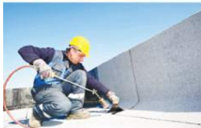
Fig. 5.2: Execution process of waterproofing works
