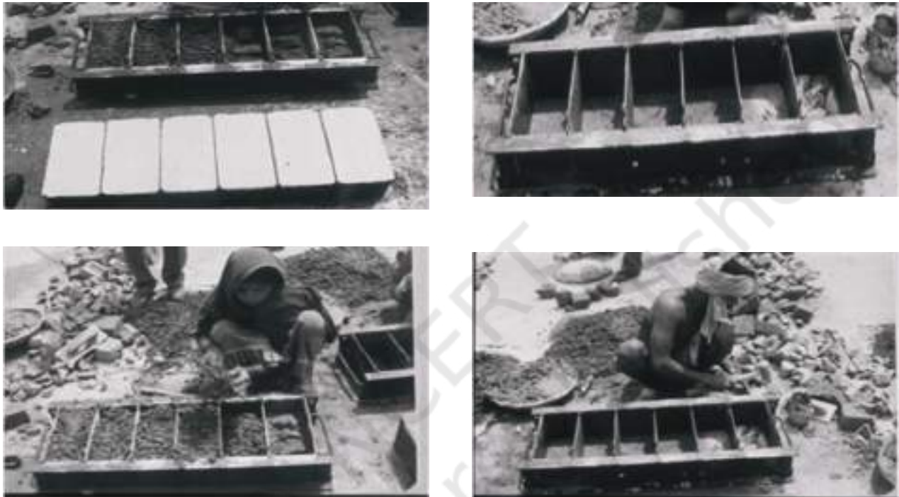
Fig. 4.8: Steps in moulding of concrete block
