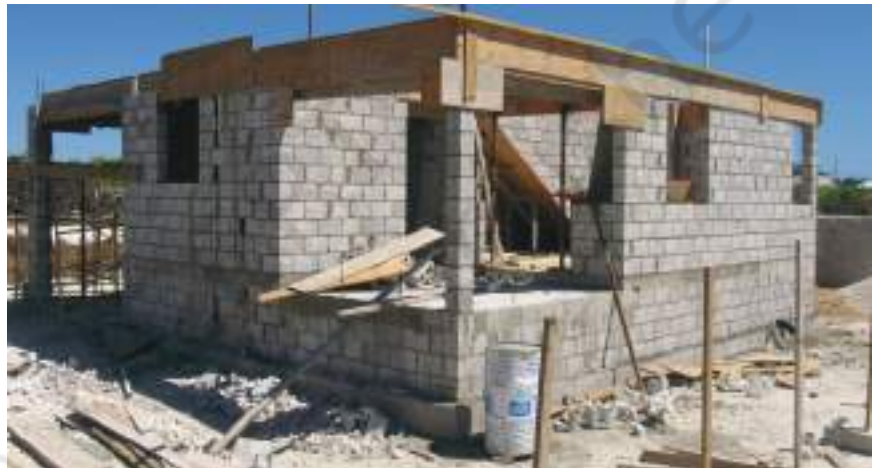
Fig. 4.12: Concrete block wall in house construction
