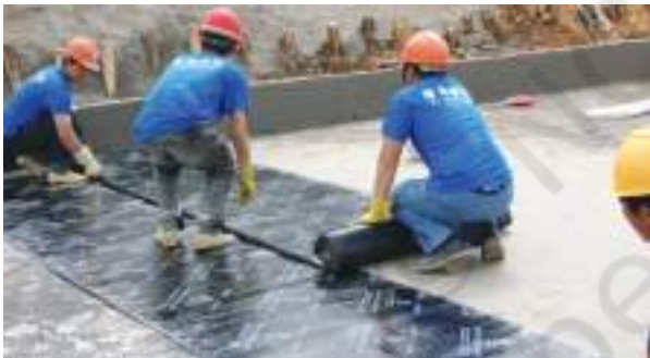
Fig. 5.14: Bituminous Membrane Laying
