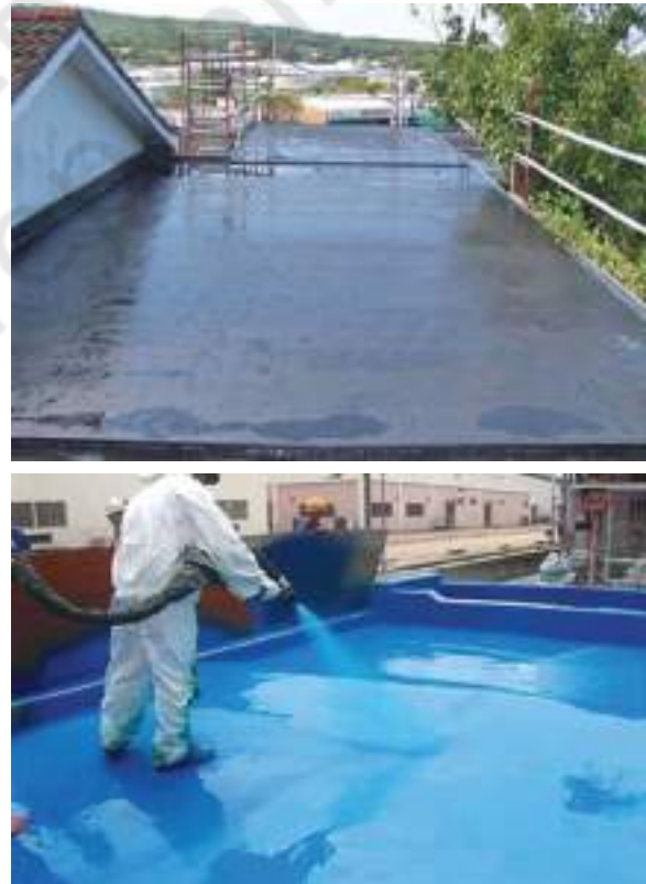
Fig. 5.17: Poly Acrylic chemical coating waterproofing
