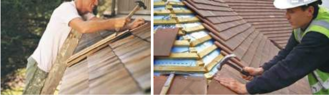
Fig. 5.18: Pre-monsoon roof repairing
