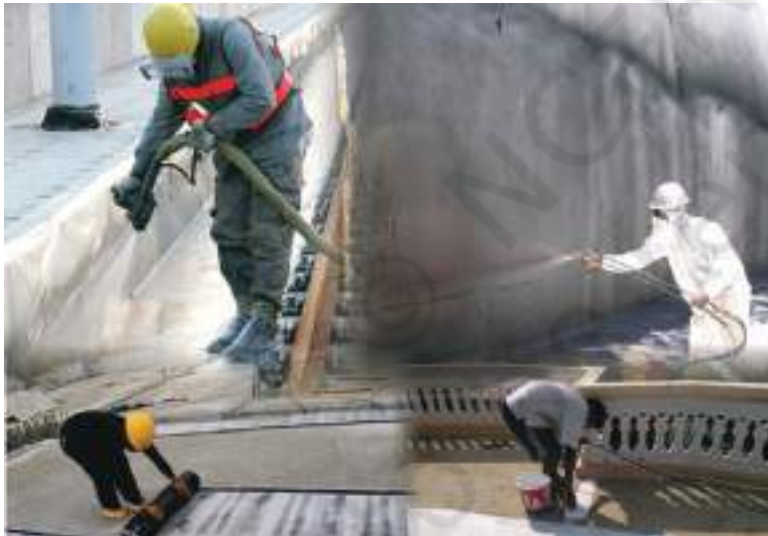
Fig. 5.1: Standard practices for waterproofing
