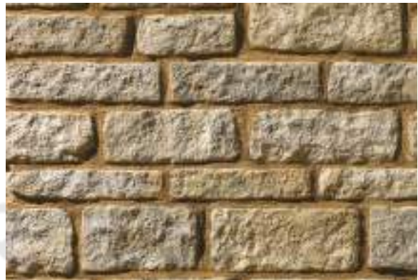
Fig. 1.17: Ashlar rough tooled masonry
