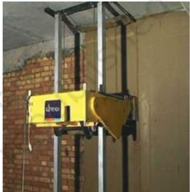
Fig. 3.2: Plastering with machine
