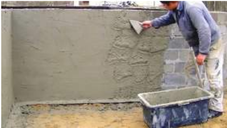
Fig. 3.3: Plastering with manual labour
