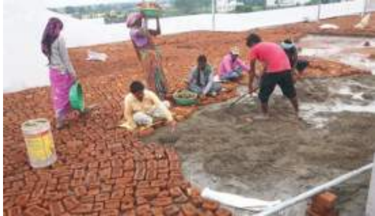
Fig. 5.16: Brick Bat coba waterproofing
