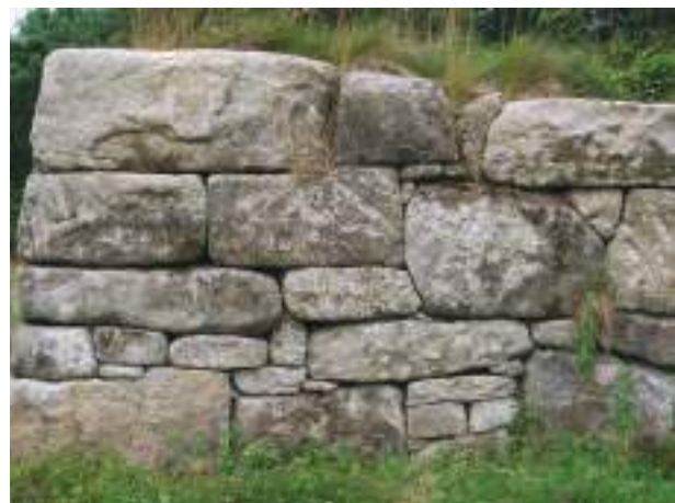
Fig. 1.12: Dry Rubble Masonry
