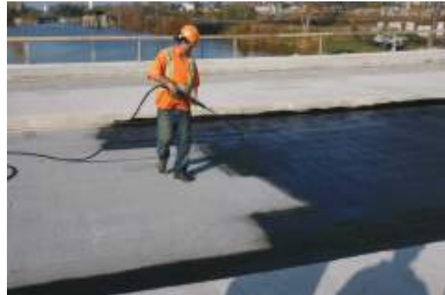
Fig. 5.9: Spraying waterproofing material
